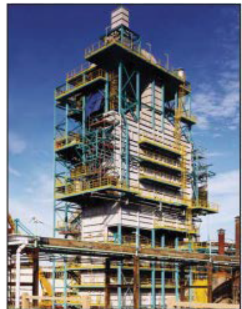
Ethylene Cracker Unit
